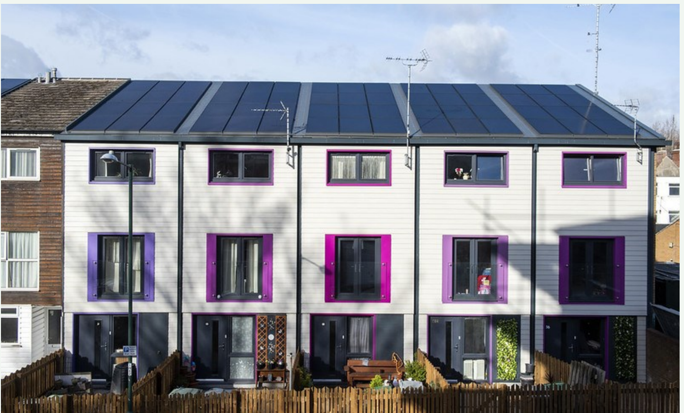
A home retrofit project in Nottingham. Photo by Tracey Whitefoot.
